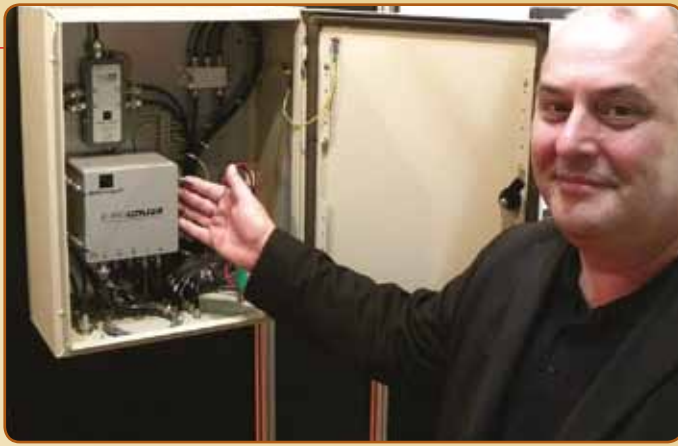
■ New at GlobalInvacom: a housing with four stacked ODU32 components that provides eight identical optical connections, capable of feeding 256 points.
